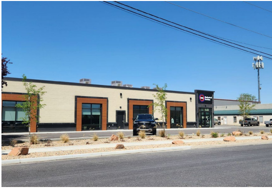
Example of drought-tolerant commercial landscaping.
