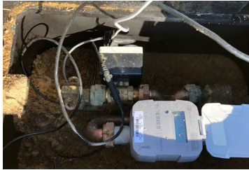
Secondary water meter that can be read digitally.
