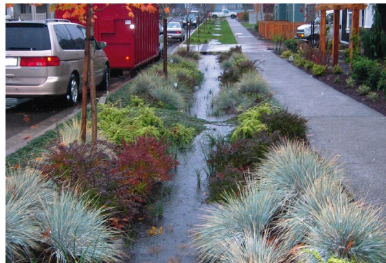
Example of bioretention in a parkstrip.
