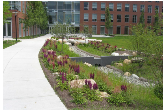
Stormwater capture with local plants.
