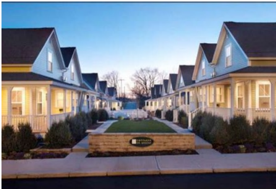
Efficient landscaping for a shared residential open area.
