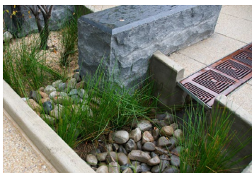
Installation of bioretention in a highly trafficked pedestrian area.
